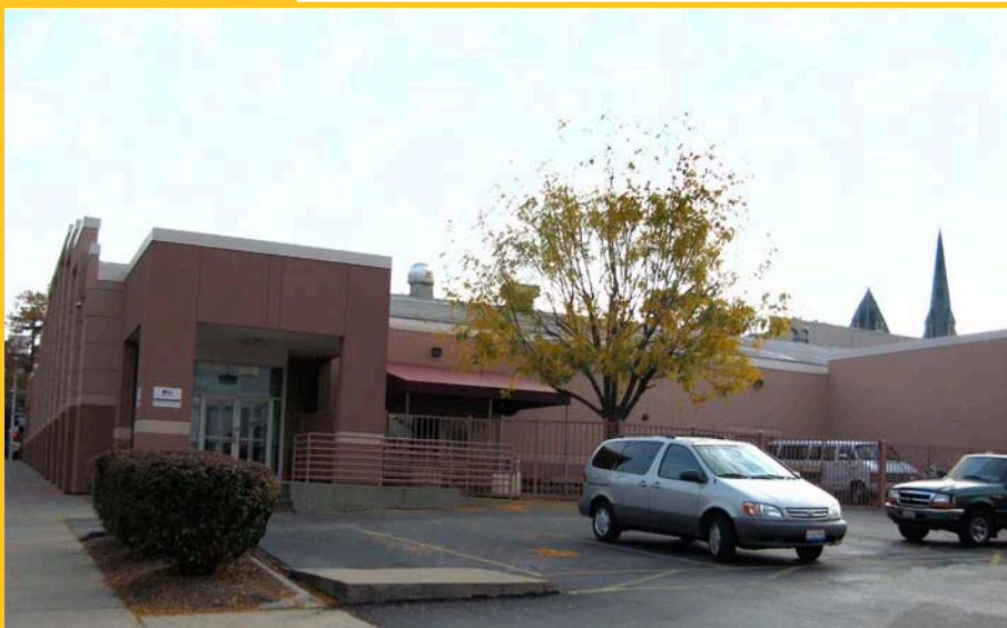
New Building, rear entrance, with additional parking and patio area
